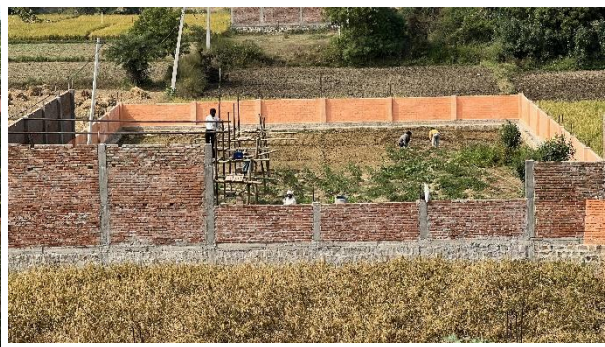
New playground (600 sqm) with drainage
